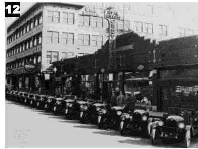
Northeast corner of 5th and Nebraska
