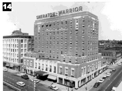
Northwest corner of 6th and Nebraska Street
