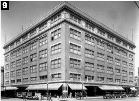
Northeast corner of 4th and Nebraska
