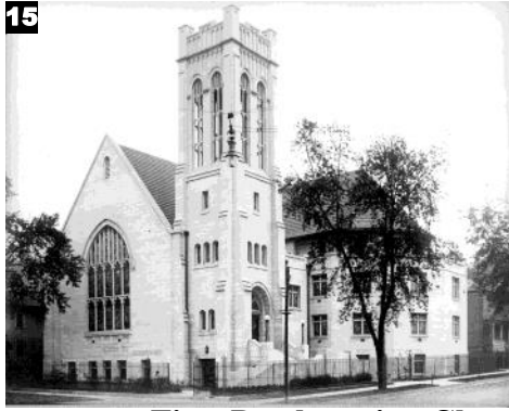
Northeast corner of 6 th and Nebraska
